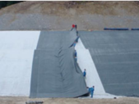
Firestone Lining Systems are based on EPDM Geomembranes, a highly flexible rubber waterproofing membrane offering numerous benefits, as demonstrated in thousands of exposed applications worldwide.
